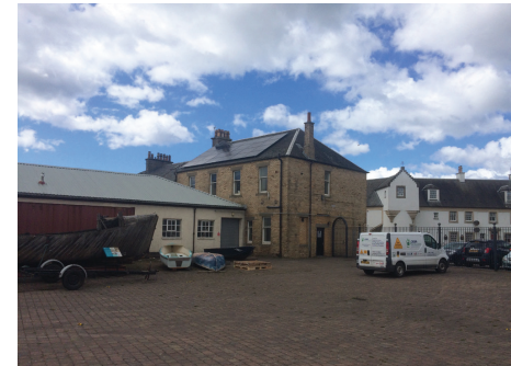
> The Scottish Maritime Museum posed a particular challenge in being very much a working building in a conservation area
